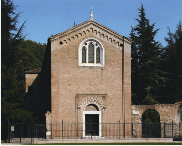
Arena (Scrovegni) Chapel
